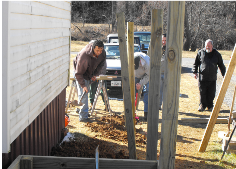
SOBER residents build handicapped access ramp to cancer survivor's home.
